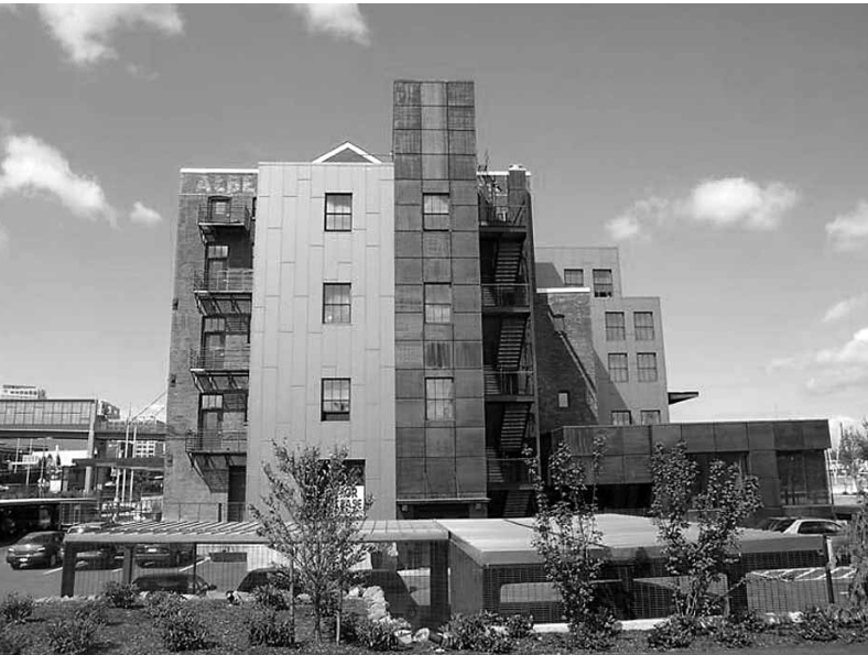
Albers Mill in Tacoma was one of the first projects in the country to use New Markets Tax Credits.
