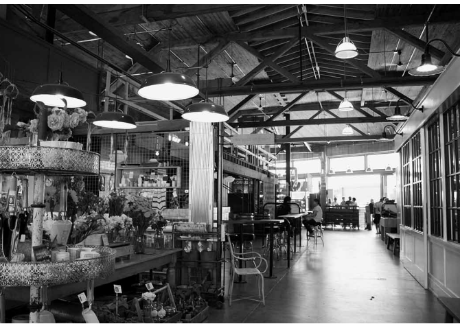
Preserving old buildings, such as the recently refurbished Melrose Market in Seattle's Capitol Hill neighborhood, provides greater green benefits over demolition and new construction. Photo by Kevin Keim, courtesy of Dunn + Hobbes.
