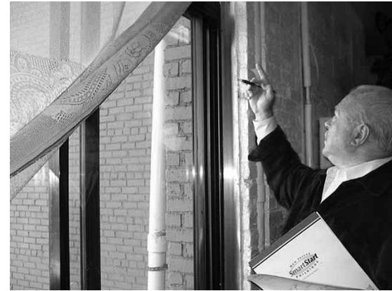
Public Service Electric and Gas Company (PSE&G) and New Jersey Housing and Mortgage Finance Agency (NJHMFA) collaborated in order to deliver energy efficiency improvements to low-income customers. Photo courtesy of PSE&G.
